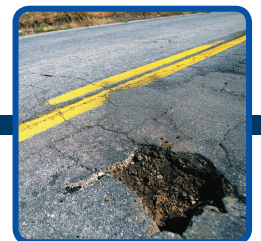
POTHoles/DAMAGED PAVEMENT
